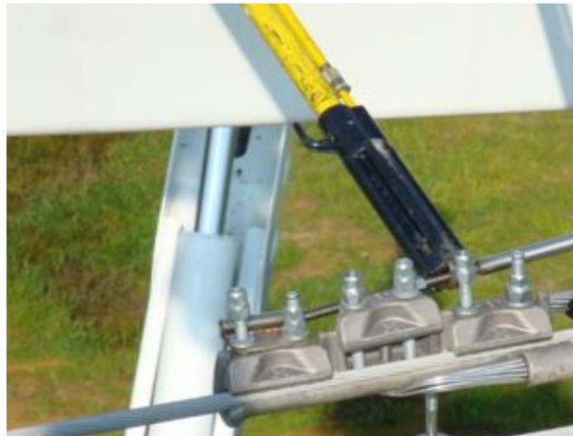
And slip the threaded ends of the Safe-T-Link Tether into each respective bracket.
